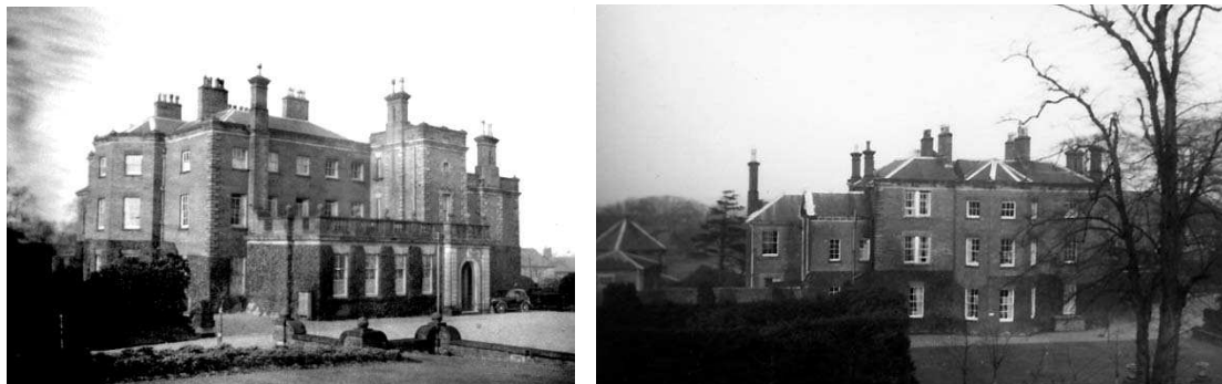
Front and rear views of Stallington Hall - photographs courtesy of William Roylance 'Roy' Mayer
